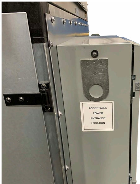
Fig. 175 — Acceptable Power Entrance Location
